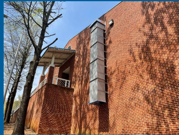
Exterior HVAC Duct Work Installed
