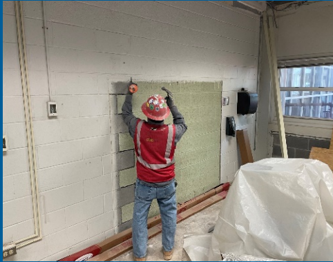
CMU Block demo for replacement infill
