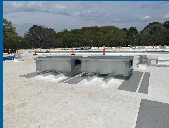
Extended HVAC curbs installed on Roof
