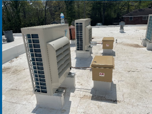
Routing condensate lines to rooftop VRF units
