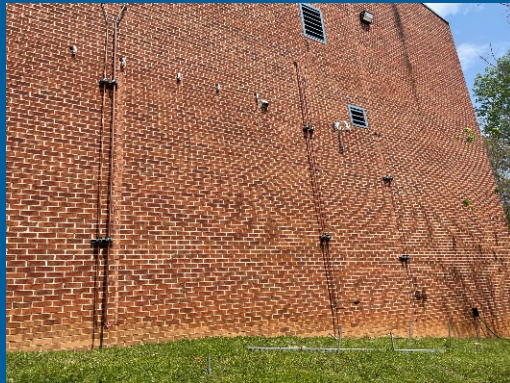
Condensate Lines installed at Gym Area
